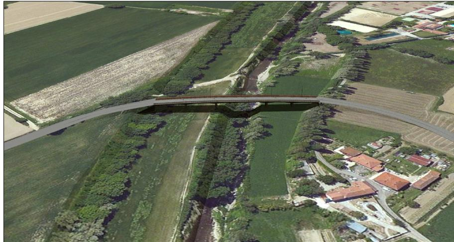
PONTE AD ARCO SU CAMPATA CENTRALE SU 2 PILE E 2 SPALLE
